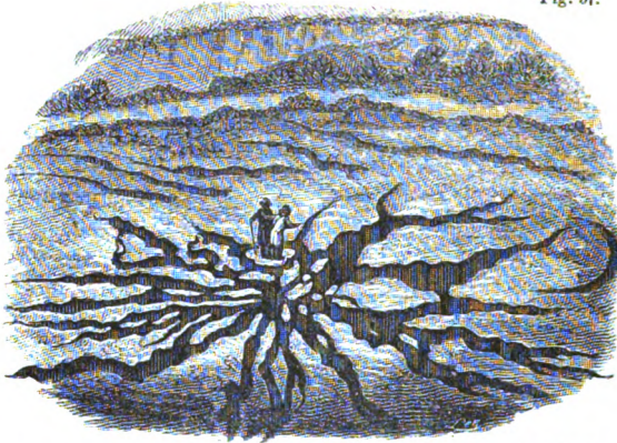
Fissures near Jerocarne, in Calabria, caused by the earthquake of 1783.
