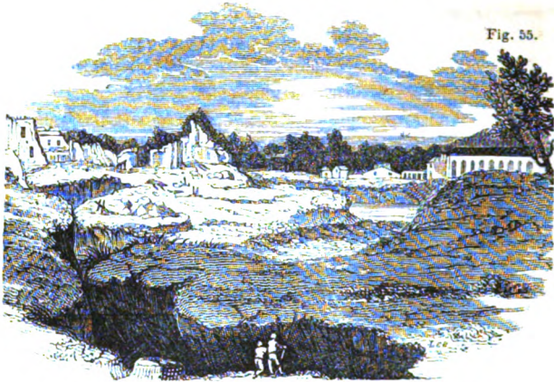
Deep fissure, near Pollistena, caused by the earthquake of 1783.
