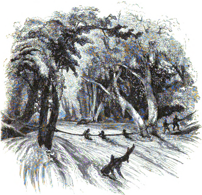
Rude Bridge over the Ovigui.
