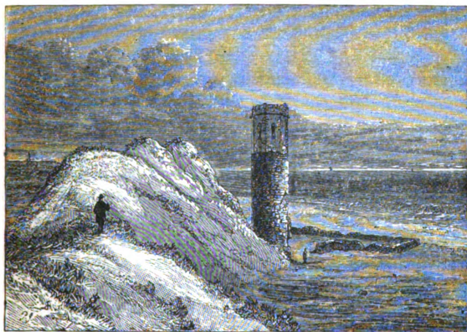
Eccles Tower as it appeared after the storm of November 1862, from a drawing by Rev. S. W. King, taken from nearly the same position as fig. 50.
