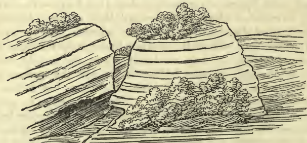
Fault in the Ravine to the right of the signal-house, Studland.
