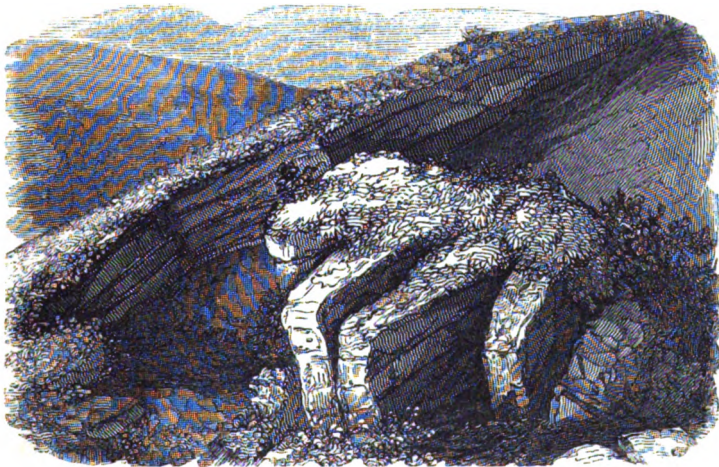
THE PALMER'S CAIRN LANDSLIP.
