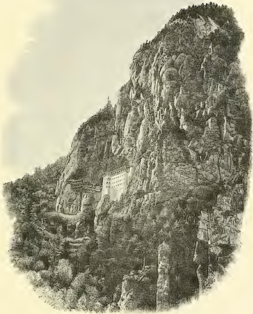
Monastery of Sumila, Stauros near Trebizond.
