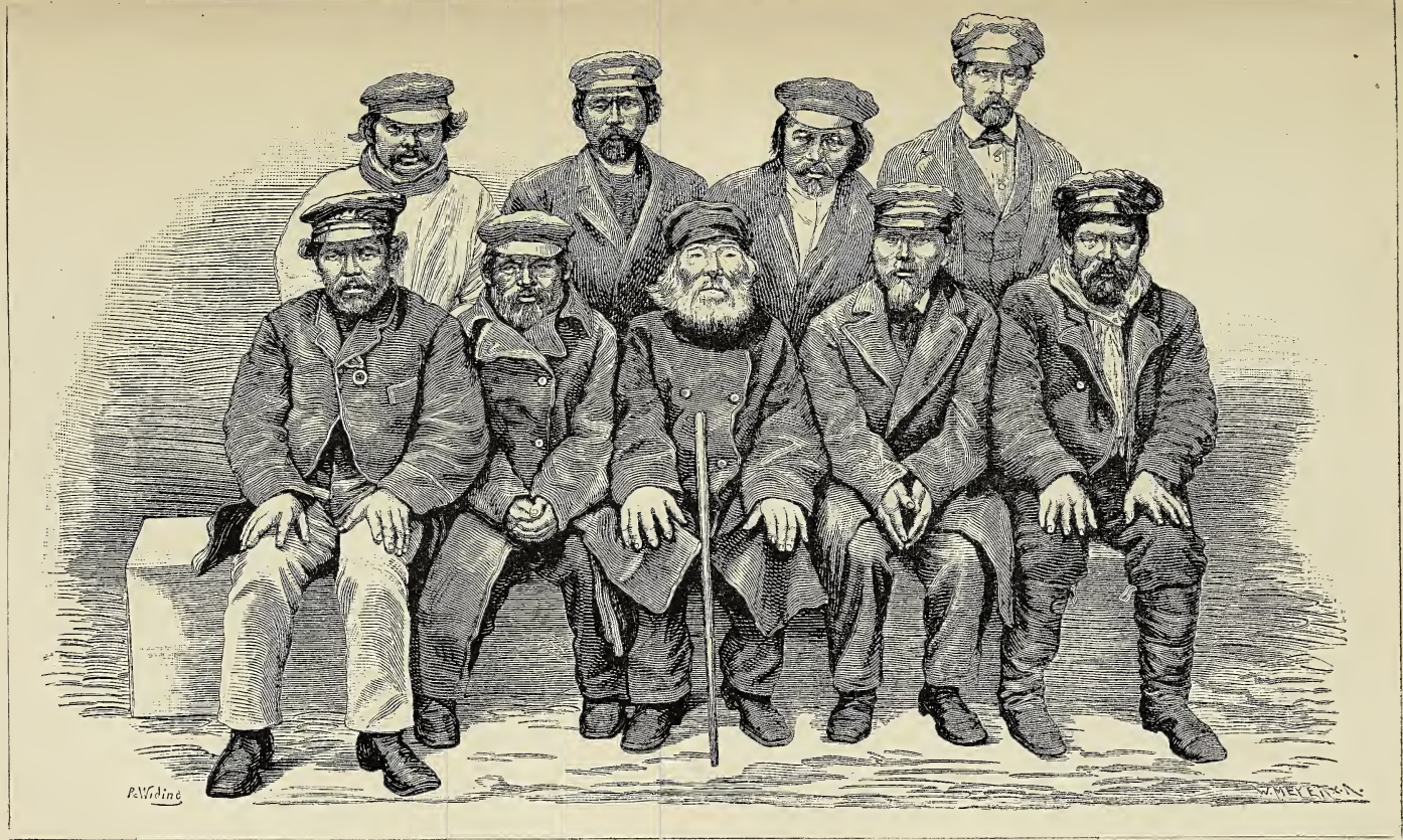
NATIVES OF BEHRING ISLAND, (After a photograph.)
