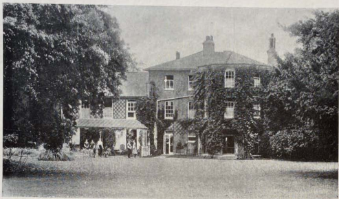
DOWNE HOUSE, DOWNE, KENT. 1907-1922
