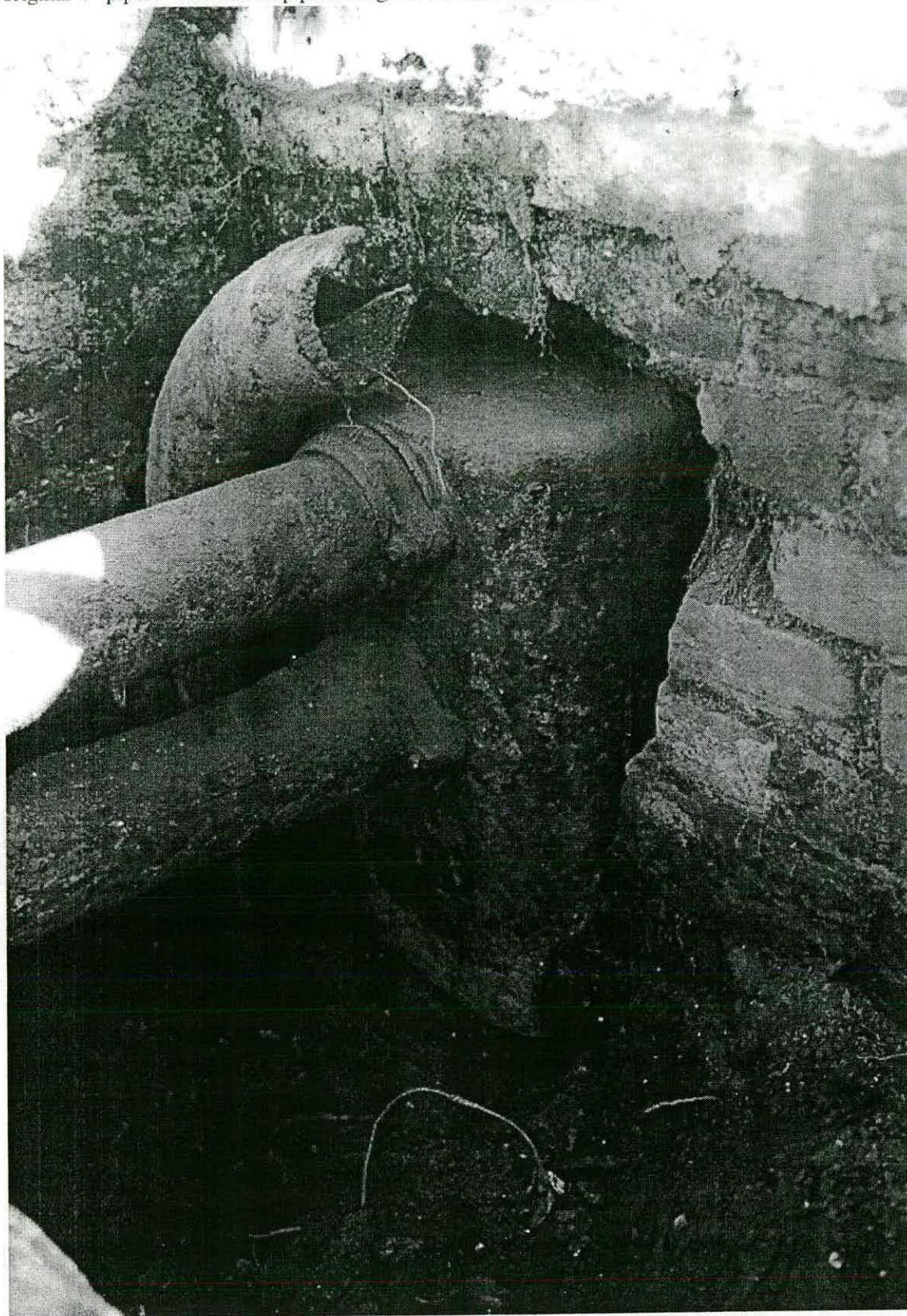
Figure 7 Back of the water jacket set in the south wall of the hothouse of 1863, with the original 4" pipes. The curved pipe belongs to the 1864 extension.
