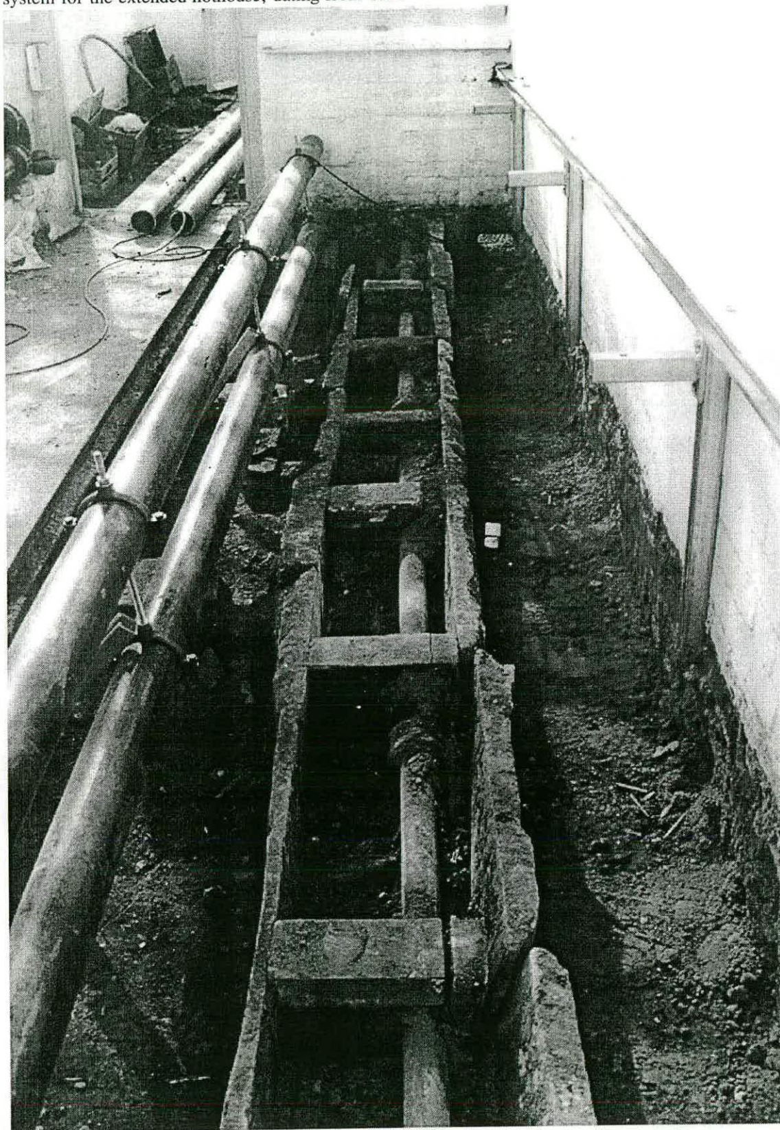
Figure 14 The channel on the north side of the hothouse for the 2" pipes, part of the heating system for the extended hothouse, dating from 1864
